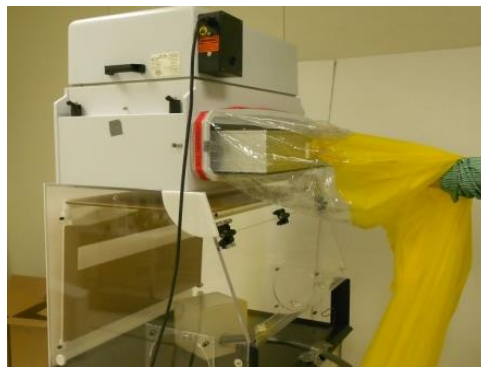
Pull primary filter forward
