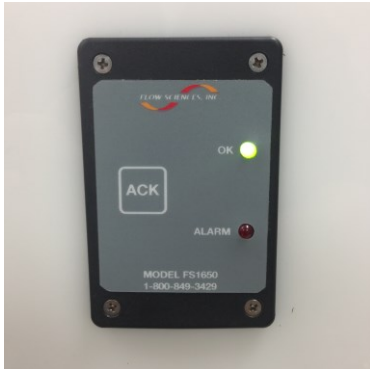
Fig. 23. Acceptable Face velocity (Green)
