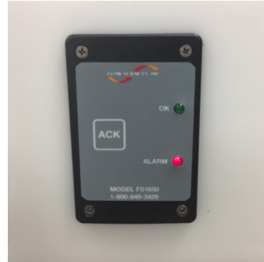
Fig. 24. Unacceptable Face Velocity (Red)
